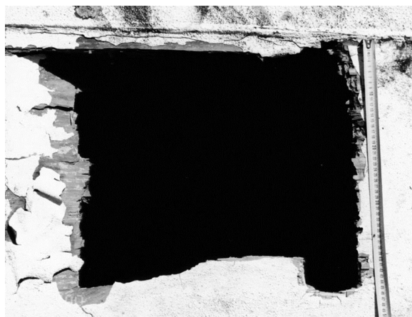
Figure 2. A photograph of the approximately 18-inch square hole in the deck of the wooden barge where the three mortar racks had broken completely through.
